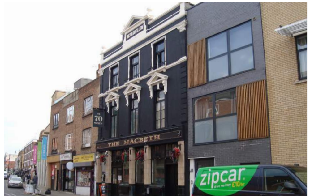
Macbeth Public House, 70 Hoxton Street (locally listed)
