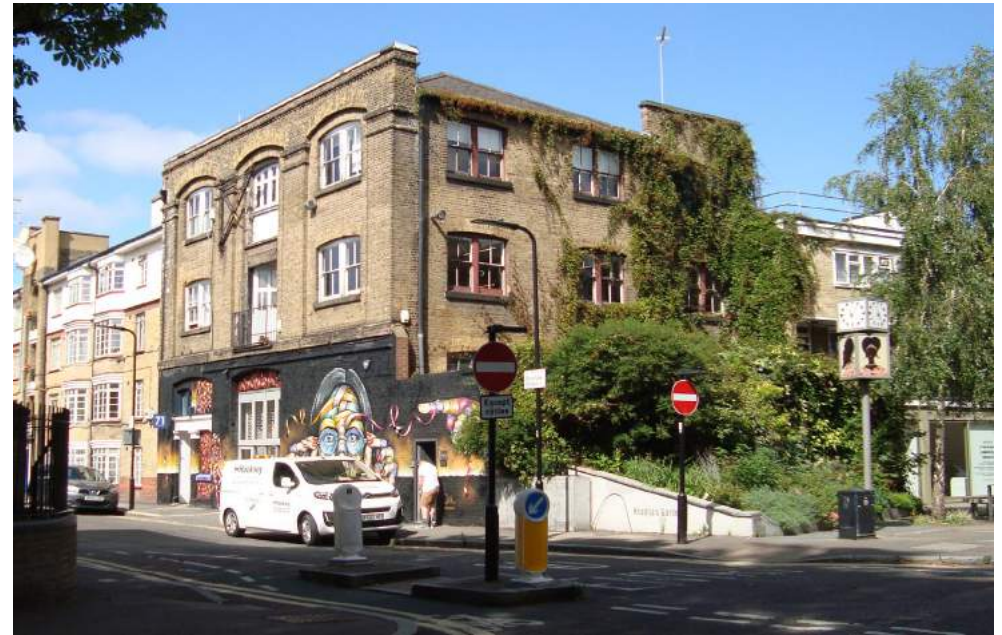
71 Fanshaw Street, demonstrating the industrial character of Hoxton
