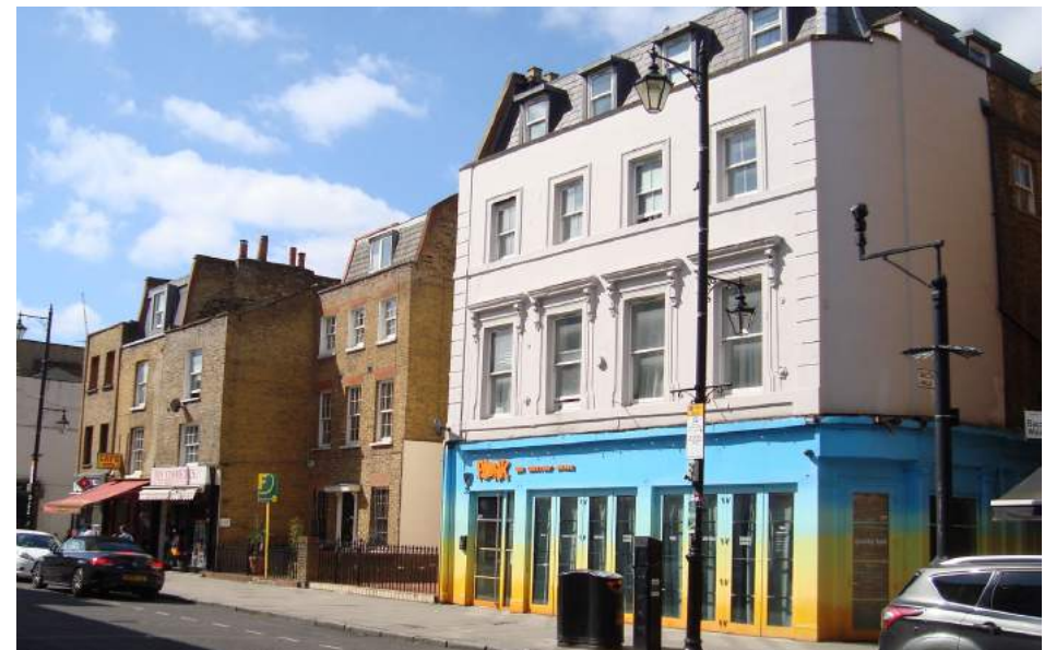
Nos 167-177 Hoxton Street, with the former Bacchus pub in the foreground
