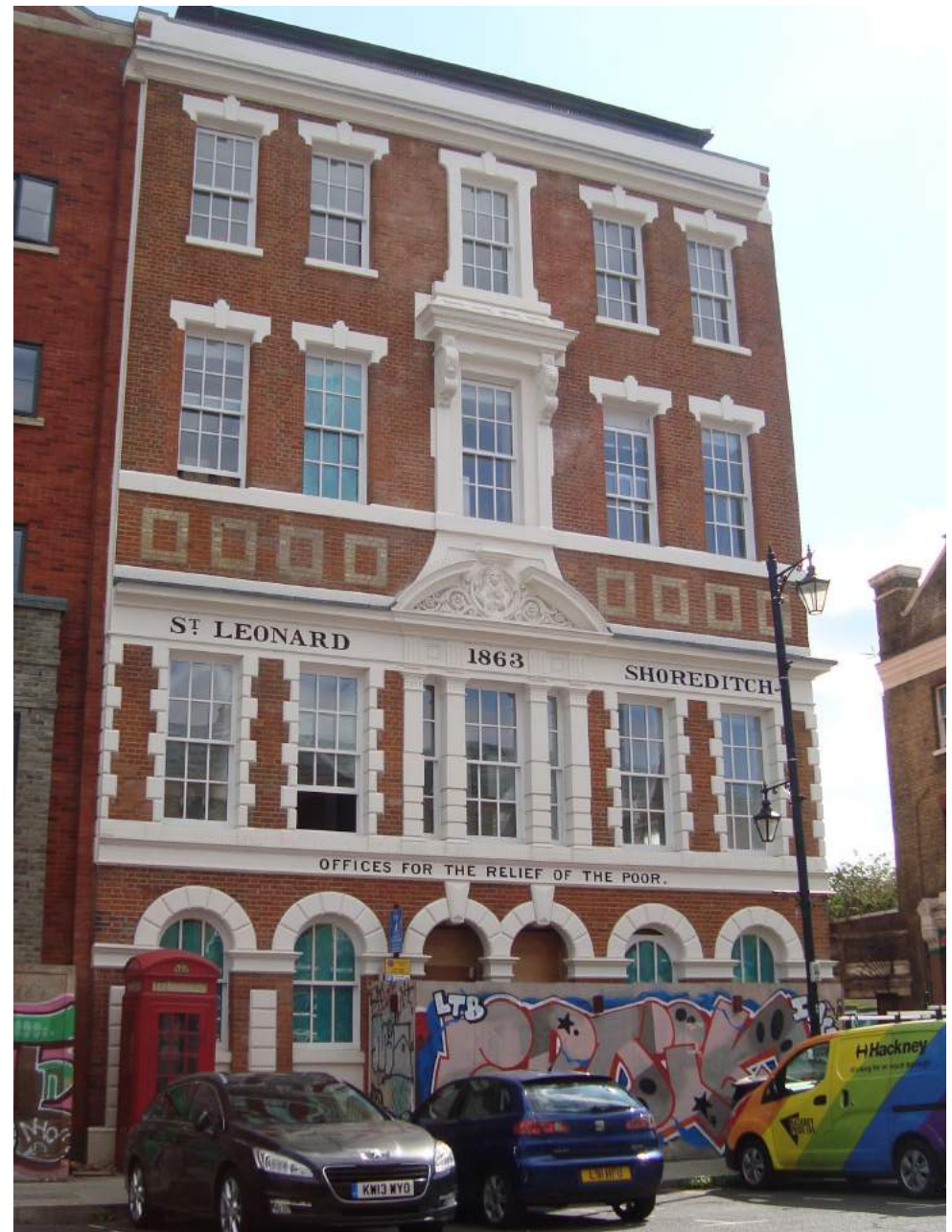
The facade of St Leonard Parish Relief Offices has been refurbished as part of a regeneration project for the wider hospital site
